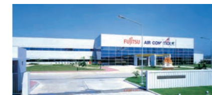
Fujitsu General (Thailand) Co., Ltd. (Thailand)
