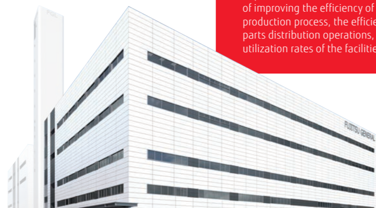
Technology research building in Japan Head office
