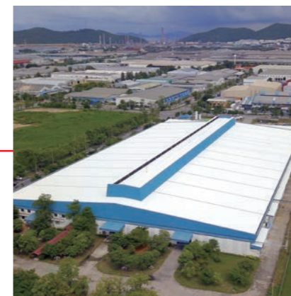
Fujitsu General (Thailand) Co., Ltd. (Thailand) Factory-2
