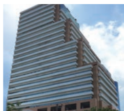
Fujitsu General (Thailand) Co.,Ltd. Bangkok Office (Thailand)
