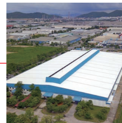
Fujitsu General (Thailand) Co., Ltd. (Thailand) Factory-2
