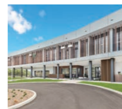
Fujitsu General (Aust.) Pty Ltd. (Australia)
