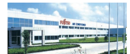
Fujitsu General (Shanghai) Co., Ltd. (China)
