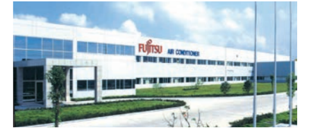
Fujitsu General (Shanghai) Co., Ltd. (China)
