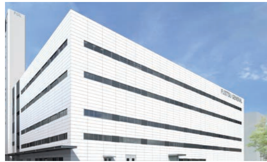
Technology research building (Japan)
