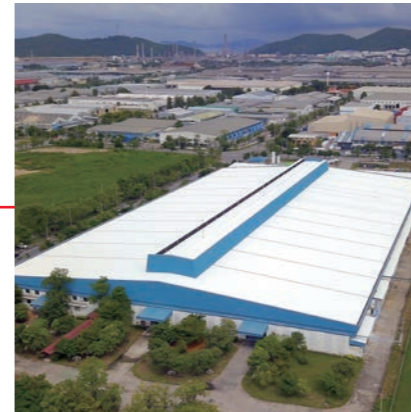
Fujitsu General (Thailand) Co., Ltd. (Thailand) Factory-2
