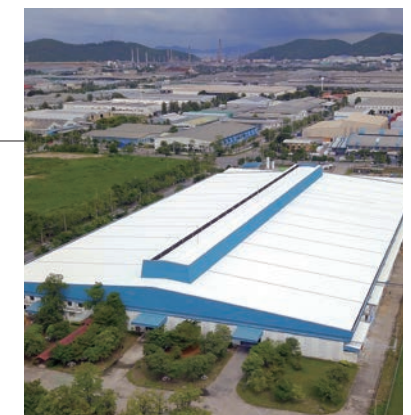
Fujitsu General (Thailand) Co., Ltd. (Thailand) Factory-2
