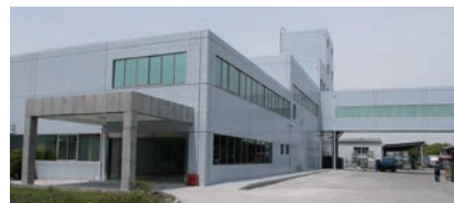
R&D center in Fujitsu General (Shanghai)
