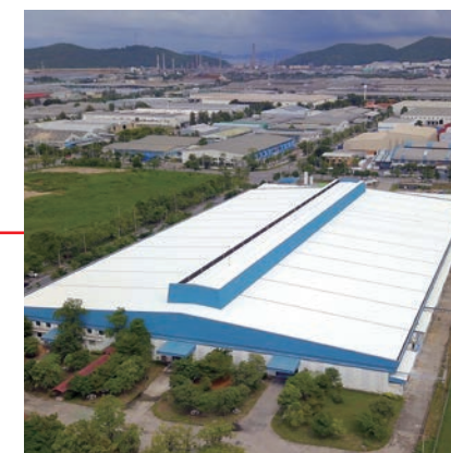
Fujitsu General (Thailand) Co., Ltd. (Thailand) Factory-2
