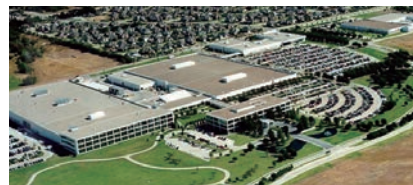
North America R&D Center (USA)
