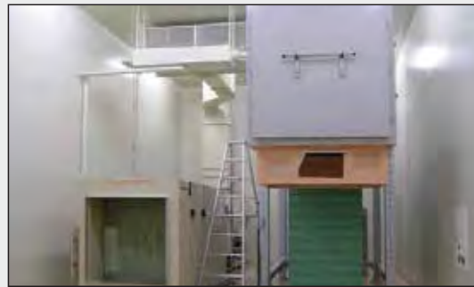
Air Volume Measurement Room
