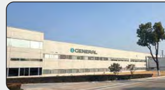
GENERAL Air Conditioning Manufacturing (Thailand) Co., Ltd.
