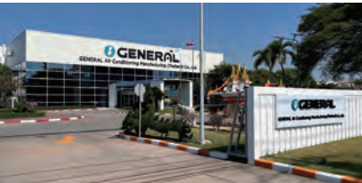
GENERAL Air Conditioning Manufacturing (Thailand) Co., Ltd.
