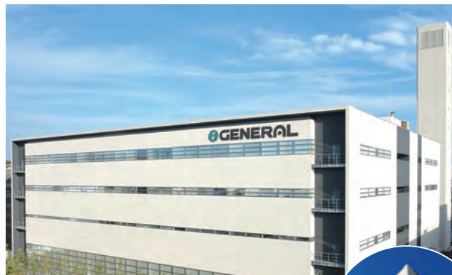
Technology Research Building in Japan Head office
