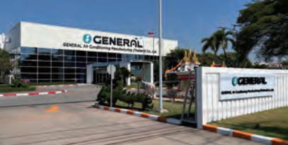
GENERAL Air Conditioning Manufacturing (Thailand) Co., Ltd.
